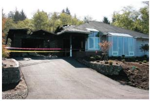
In rural Oregon, these photos show the before and after of an accidental fire that started in the garage. This home was constructed with Insulated Concrete Forms and the partition wall between the garage and the home protected the living spaces. This fire raged for 35 minutes prior to the fire department arriving.<sup>3</sup>
